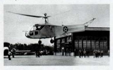
The R-4A was a small, 180-horsepower machine with a cruising speed that barely rivaled the automobile. The R-4A differed from earlier rotary wing aircraft designs. It incorporated a single main rotor above its cockpit and a smaller anti-torque tail rotor. Its 35 foot, 5 inch fuse-lage was tapered behind the cockpit. With the exception
