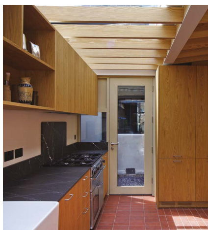
Ketley's Staffordshire Red quarry tiles laid in the new kitchen extension to the Grade II listed Van Gogh House in London.
