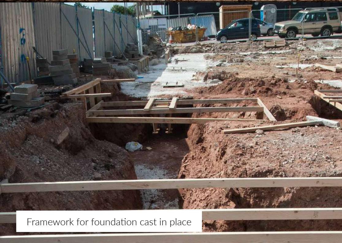
Preparing foundations for steel framework
