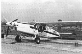
The Swiss-built Pilatus Porter was a versatile little plane specially designed to land on very short, unprepared strips. Continental Air Services used them in Laos during the latter 1960s.
