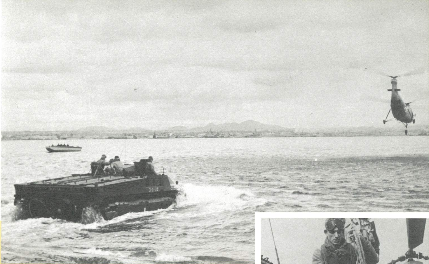
The H-21 tow helicopter moves LVT, which weighs 23,350 pounds off the beach and into the water, demonstrating its ability to clear congested beachheads of abandoned or disabled equipment.
