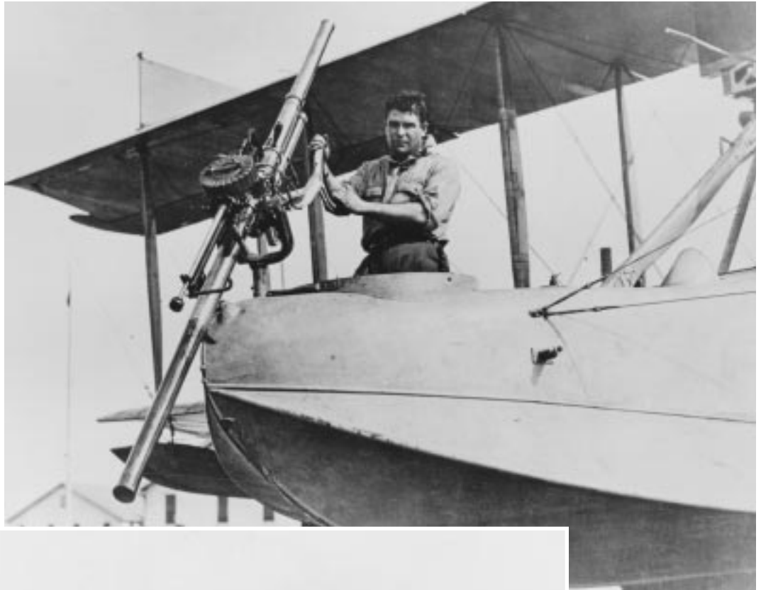
Davis recoilless ASW gun, mounted on H-1 1053766
