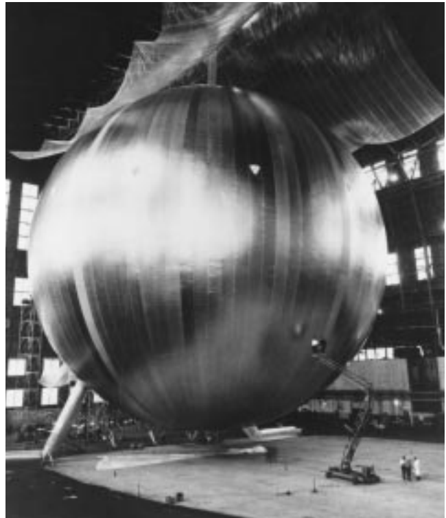
Echo II test at Lakehurst 1143455
