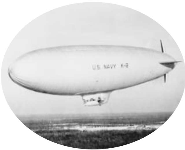
The non-rigid airship K-2, prototype for World War II LTA fleet 1053773
