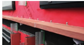
RSM - CAVITY BARRIER FOR RAINSCREEN FACADE SYSTEMS
