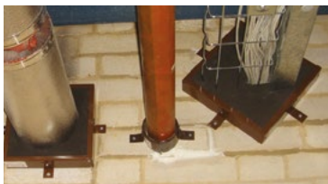
SERVICES THROUGH COLLARS & MULTI PURPOSE BOXES
