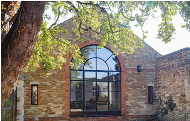
An exterior arched steel window and doors create that wow factor. Image courtesy of Squib Photography/Three Spires Glass
