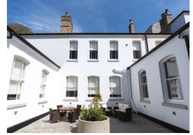
The lime rendered walls and stone window sills of this exterior courtyard feature Ecopro Silicate Masonry Paint.
