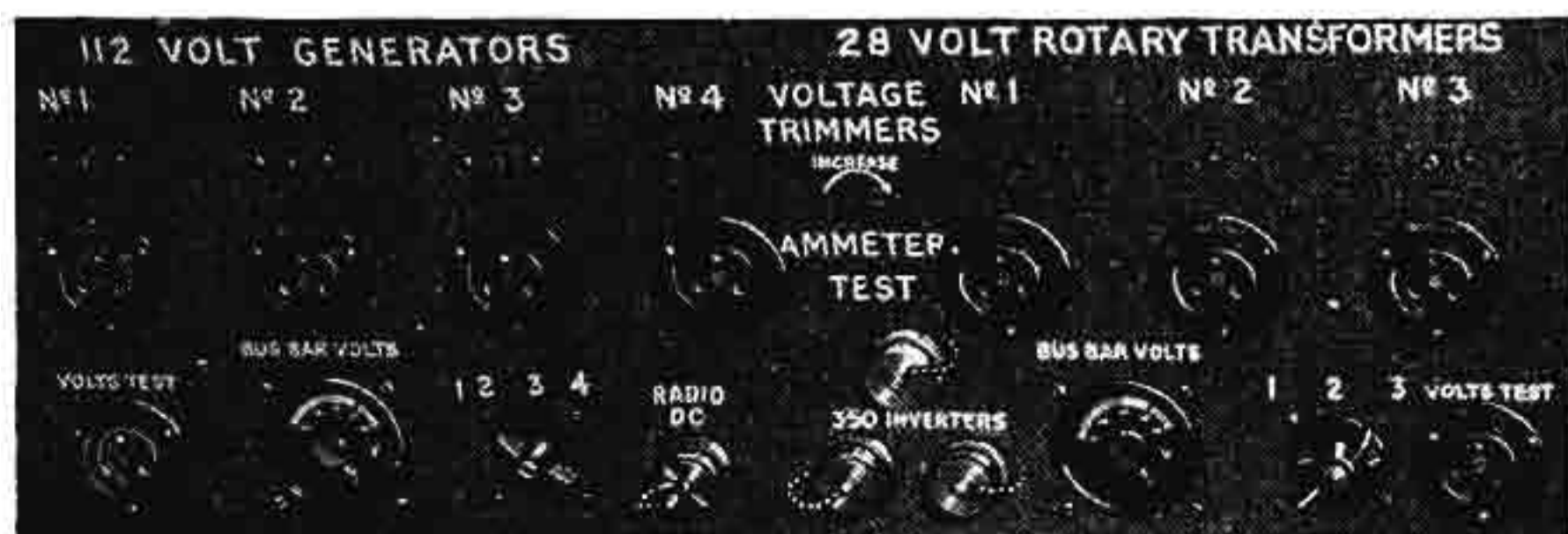
Fig. 6 Voltage trimmer panel
