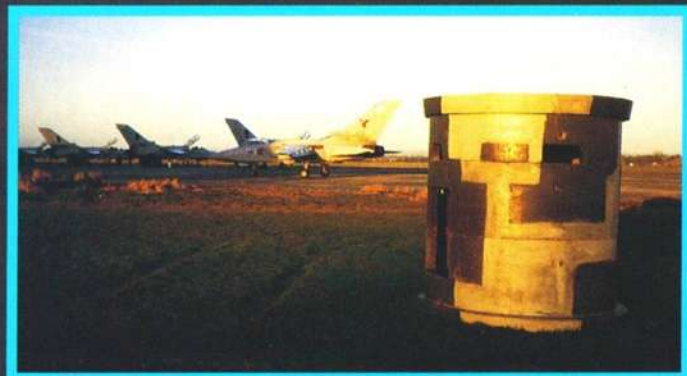
No, not a Tardis, but a Yarnold Bunker. RAF Leeming's answer to the traditional earth and sandbag bunker.
