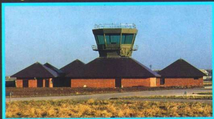
RAF Leeming's new control tower, nicknamed the Happy Eater after its A1 neighbours.
