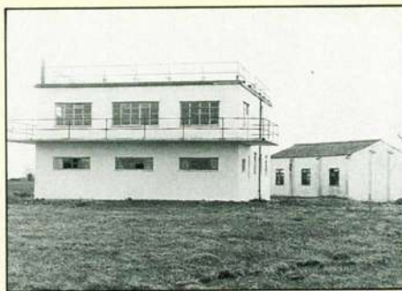
War-time style control tower with garage for a fire tender or ambulance.
