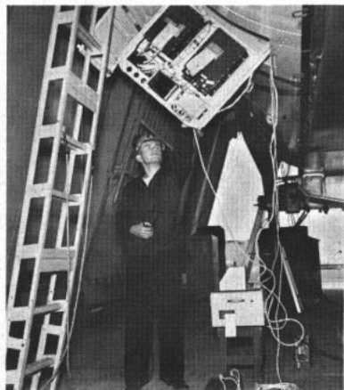
TEST equipment is connected to telemetry package in Thor booster.
