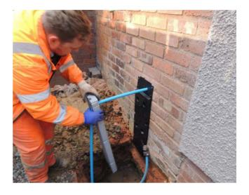
INSUduct only requires one simple core drilled hole through the wall, at an appropriate point to connect with the internal plumbing. This enables most water supply replacements to be completed within a couple of hours, without the traditional mess and disruption to the householders or occupiers. There is also little impact to the exterior appearance of the property, as the INSUduct system provides a neat, clean finish to the job.
