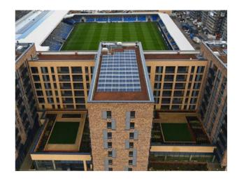
sustainable development. The 'blue roofs' will be able to hold up to 1 million litres of water after intense rainfall, which will be released slowly back into drainage systems, mitigating urban flash flooding.
