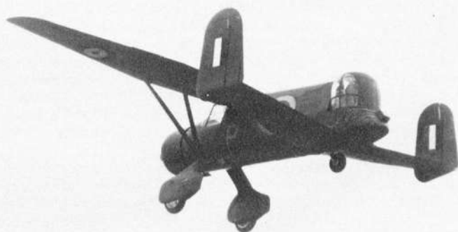
Two extreme modifications of the Lysander with the testing of which the author was concerned — (above) with the Stieger monospar wing fitted by Blackburn Aircraft, and (below) with Delanne tandem wing layout and a tail turret.
