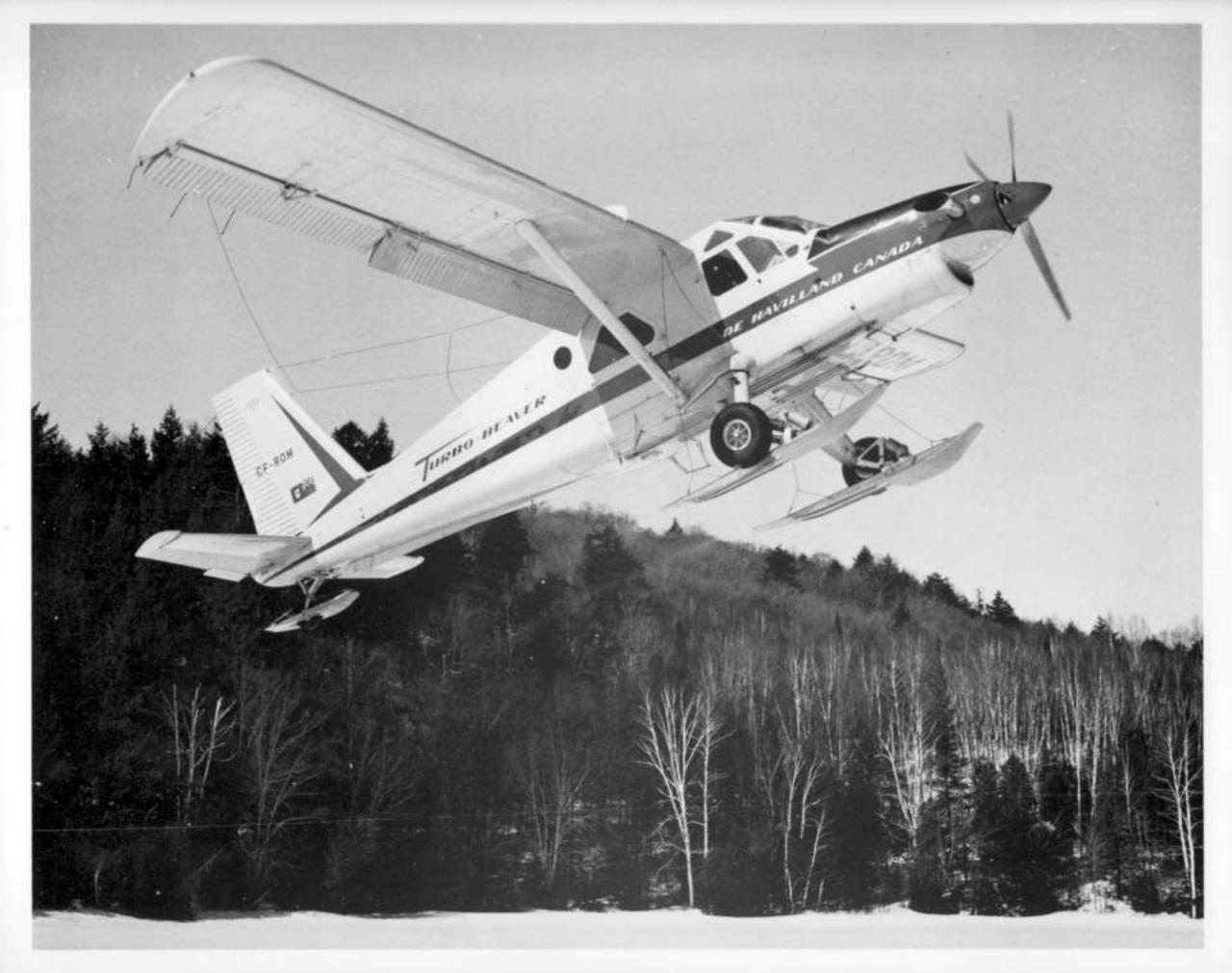
De Havilland Canada entered the jet age in 1960 with the development of the *DHC-2 Mk III Turbo-Beaver*. A lighter, more powerful PT6A-6 gas turbine engine replaced the former piston engine, giving the Beaver greater work efficiency and increased payload.
