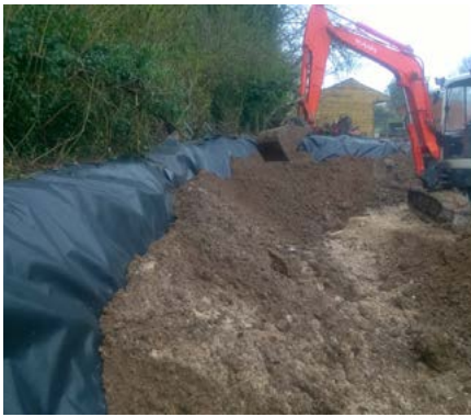
Figure 3: Knotweed Excavation with Installation of Root Barrier
