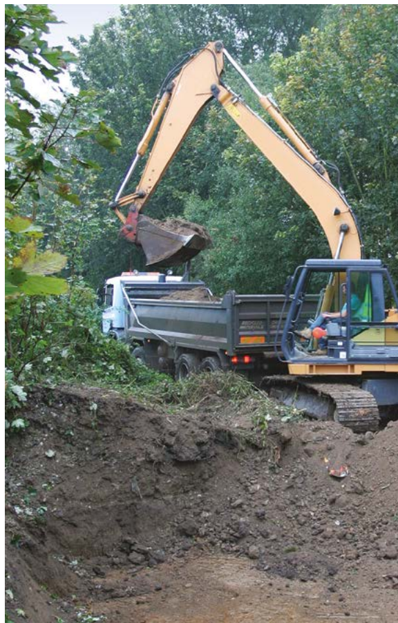
Figure 4: Dig and Dump
