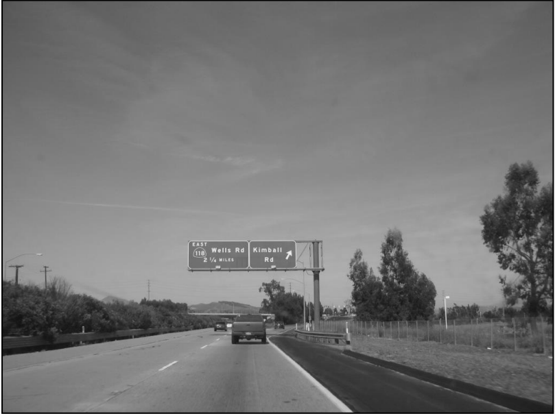
The exit to Kimball Road off Highway 126, June 2011.
