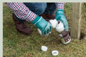
Post in position; mix the two parts.
