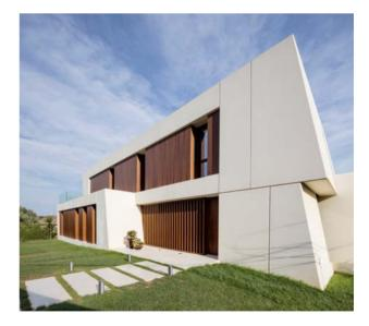
Concerning the construction system, a concrete structure is proposed that models the house from the foundations to the roof. To ensure adequate comfort, the house is fully waterproofed and insulated, covering the entire envelope with a ceramic skin.
