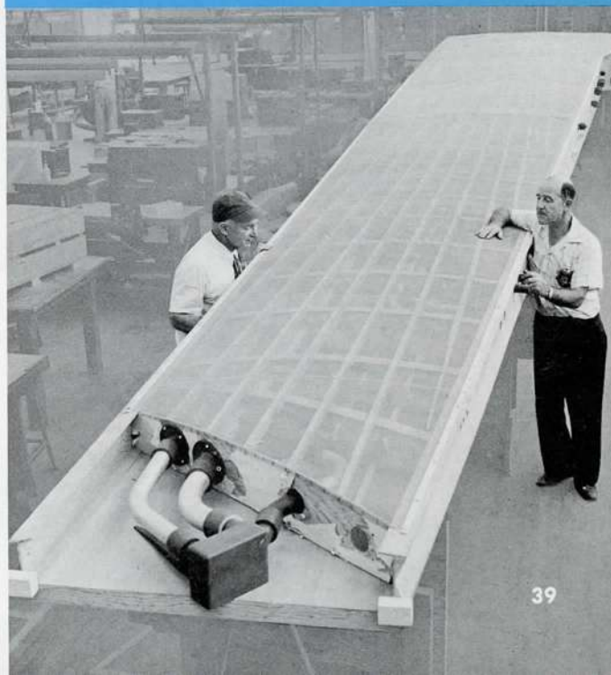
Full-scale structural mockup of wing box section provides pattern for "880" wing fabrication.
