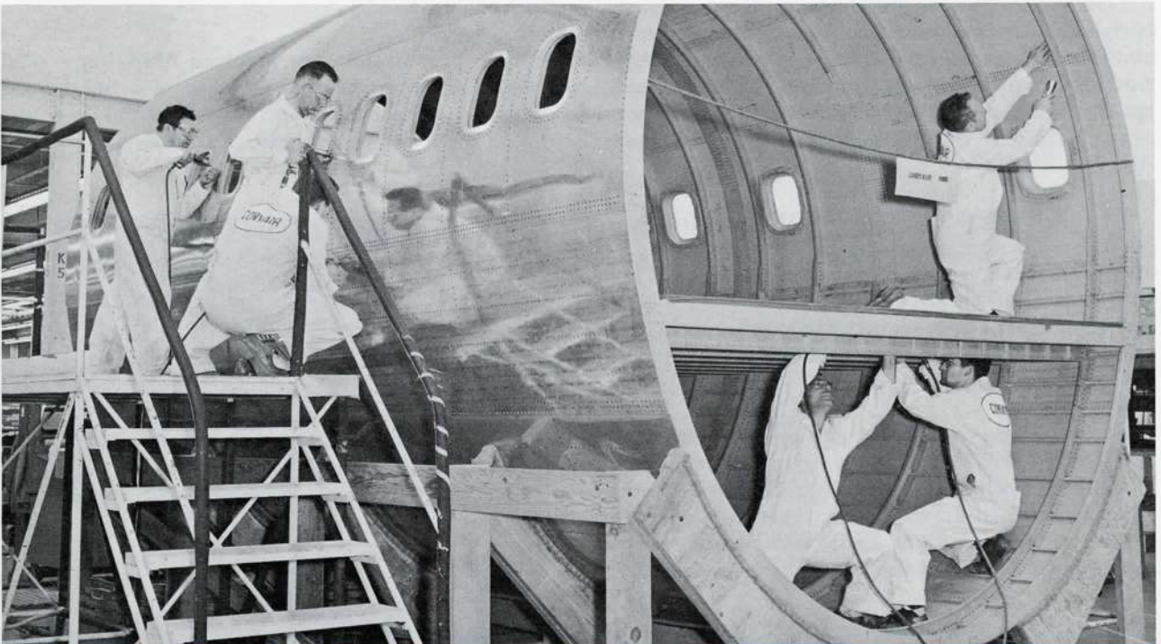
A specimen section of the "880" cabin, later to be subjected to strenuous fail-safe tests, nears completion.
