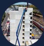
Lift & Stair Cores
