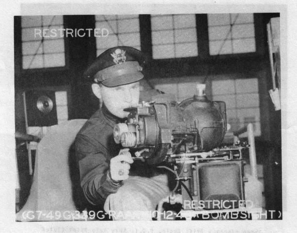
Swing on sighting over trail plate for approximate sighting by holding Auto Pilot clutch and moving sight by gripping Course Knobs.
