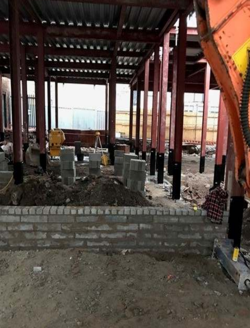
Brickwork is being prepared to lay the ground floor slab in readiness for Timber Frame erection.
