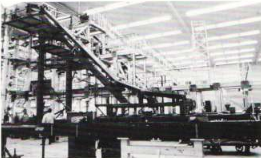
Major assembly jig for wing
