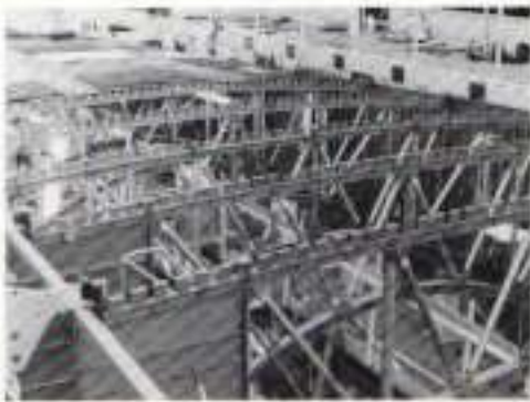
Frame and bottom skins in primary fixture
