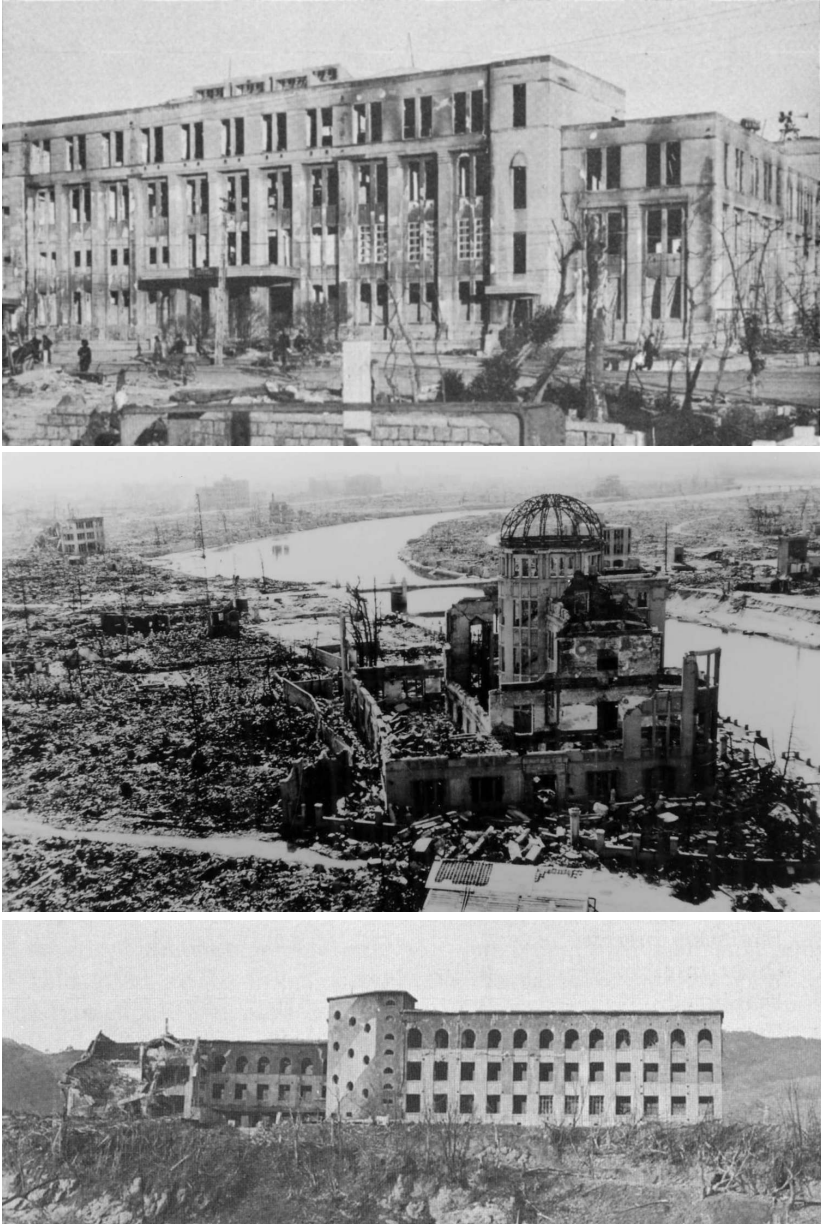
Figure 5.3 Three of many burnt-out buildings that according to various studies [83, 84] yielded pristine tiles or bricks suitable for measurement of \gamma -ray dosage by thermoluminescence. Top: Hiroshima City Hall; center: Hiroshima Prefectural Industrial Promotion Hall (now commonly called the ‘Atomic Bomb Dome’); bottom: Shiroyama elementary school in Nagasaki.
