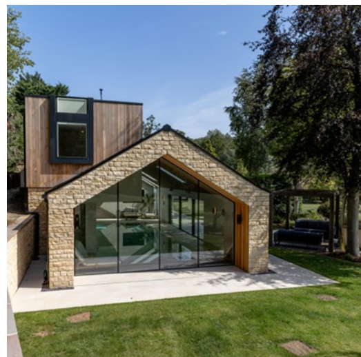
38 Swimming Pool Glazing in North Yorkshire - Old High Mill is a private leisure wing and pool hall extension to an existing home.
