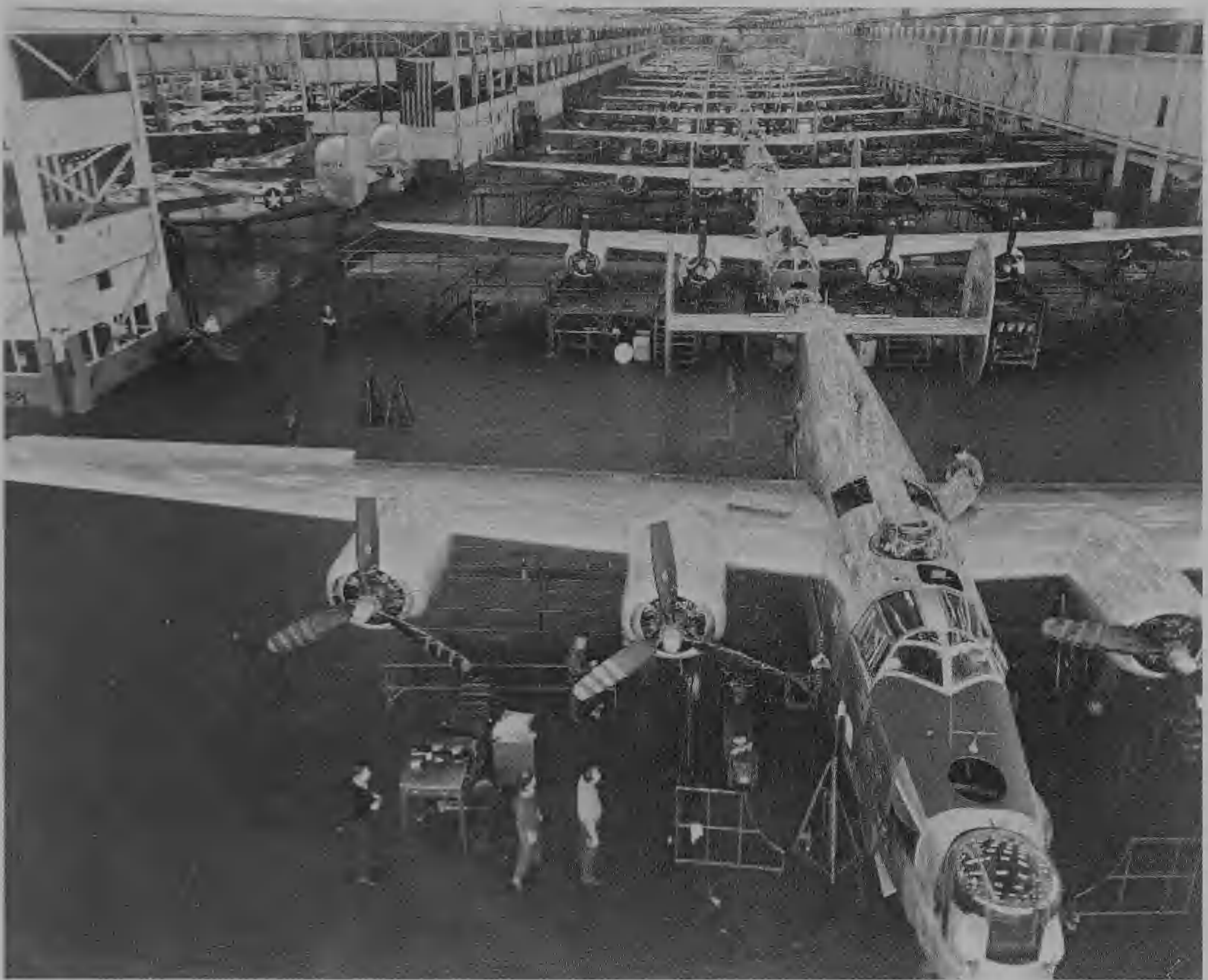
Five plants turned out B-24 Liberators during the Second World War. The Ford Motor Company of Dearborn, Michigan, built B-24H/J/L/M models in a plant covering 3,700,000 sq. ft at Willow Run. Here, some of the 1,677 B-24Ms with Emerson nose turrets are coming off the assembly lines. The serial number on the tail of the B-24 (middle) is spurious. (Ford Archives)
