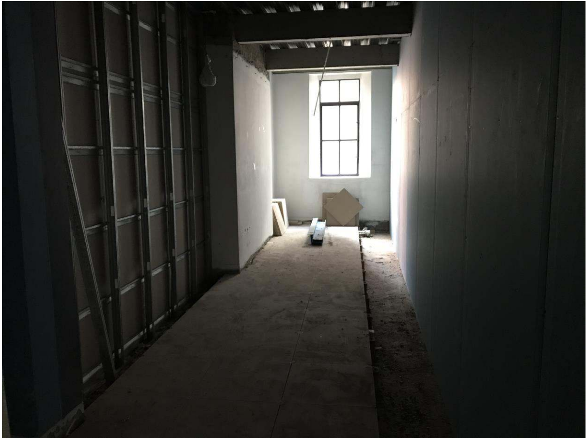
First floor party walls
