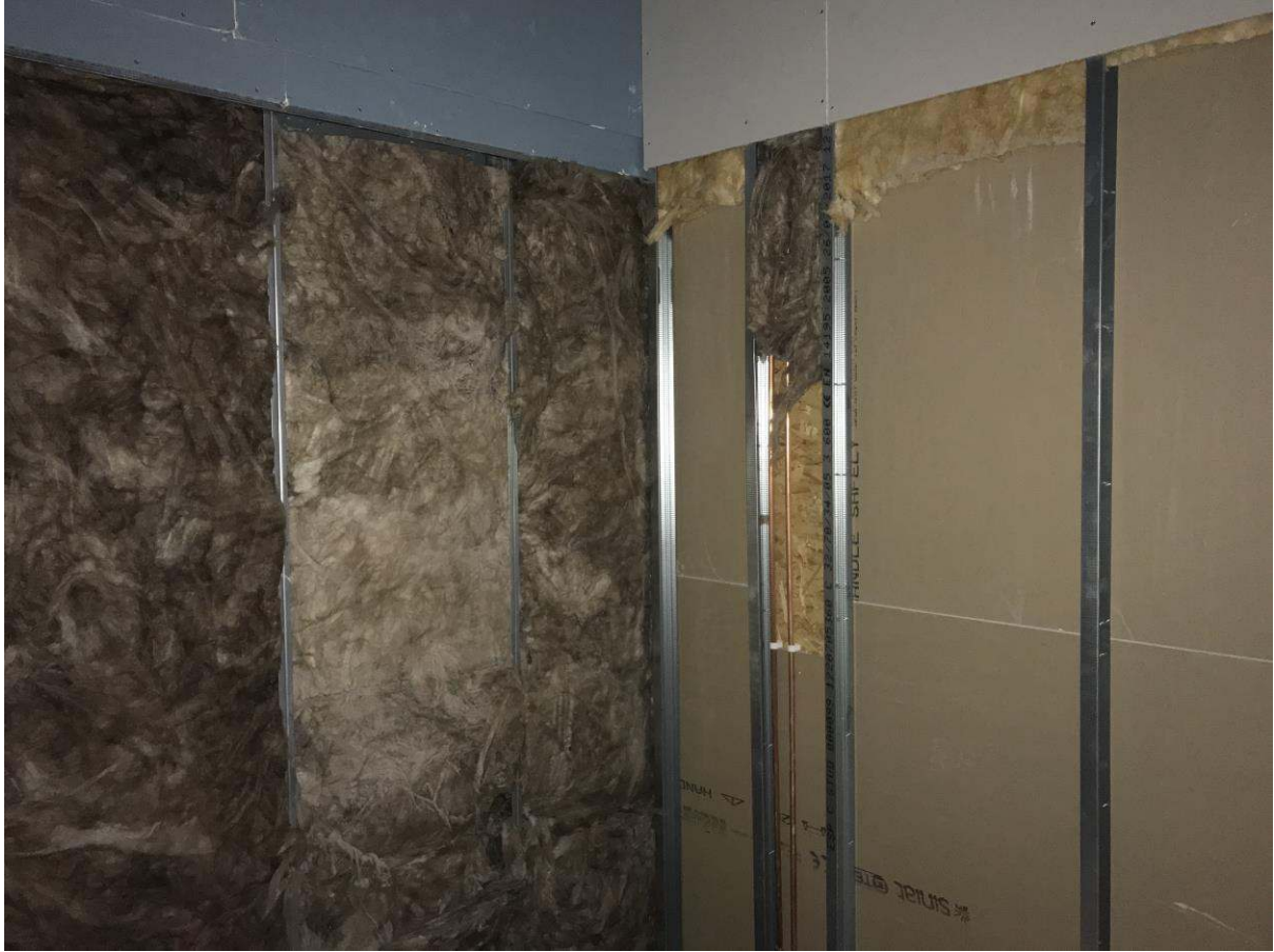
Second floor apartment M&E first fix, party wall insulation
