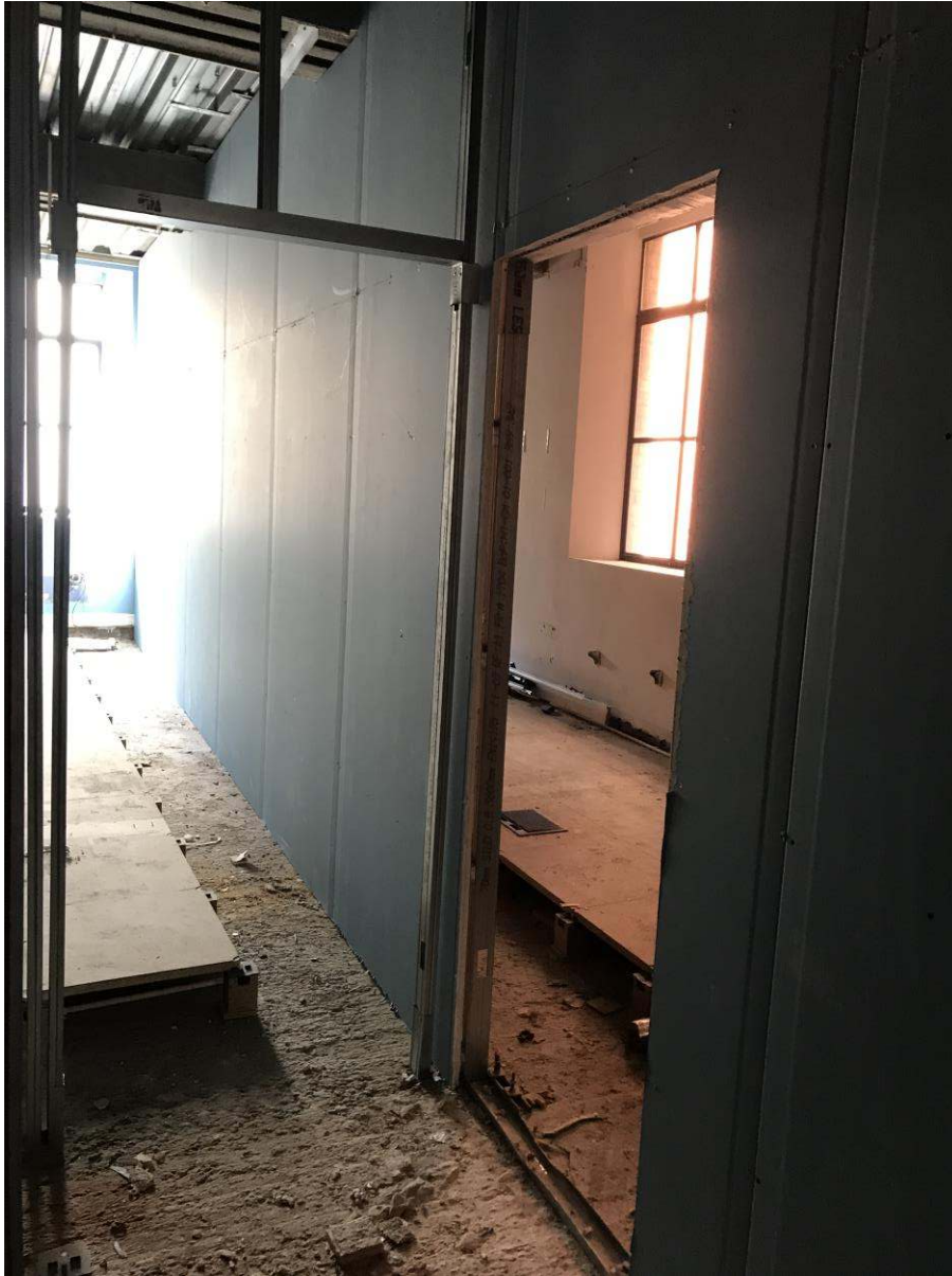
First floor party walls
