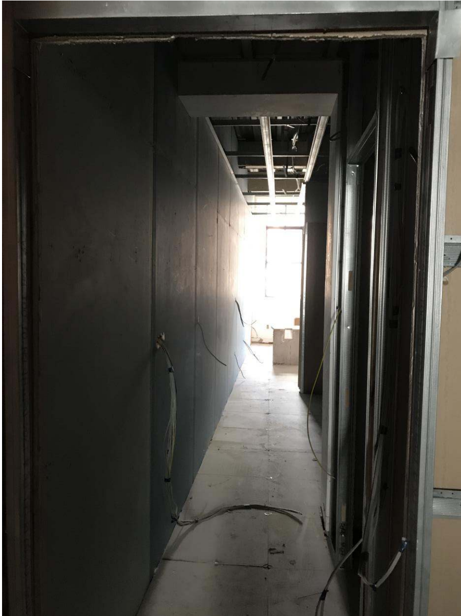
Second floor apartment M&E first fix
