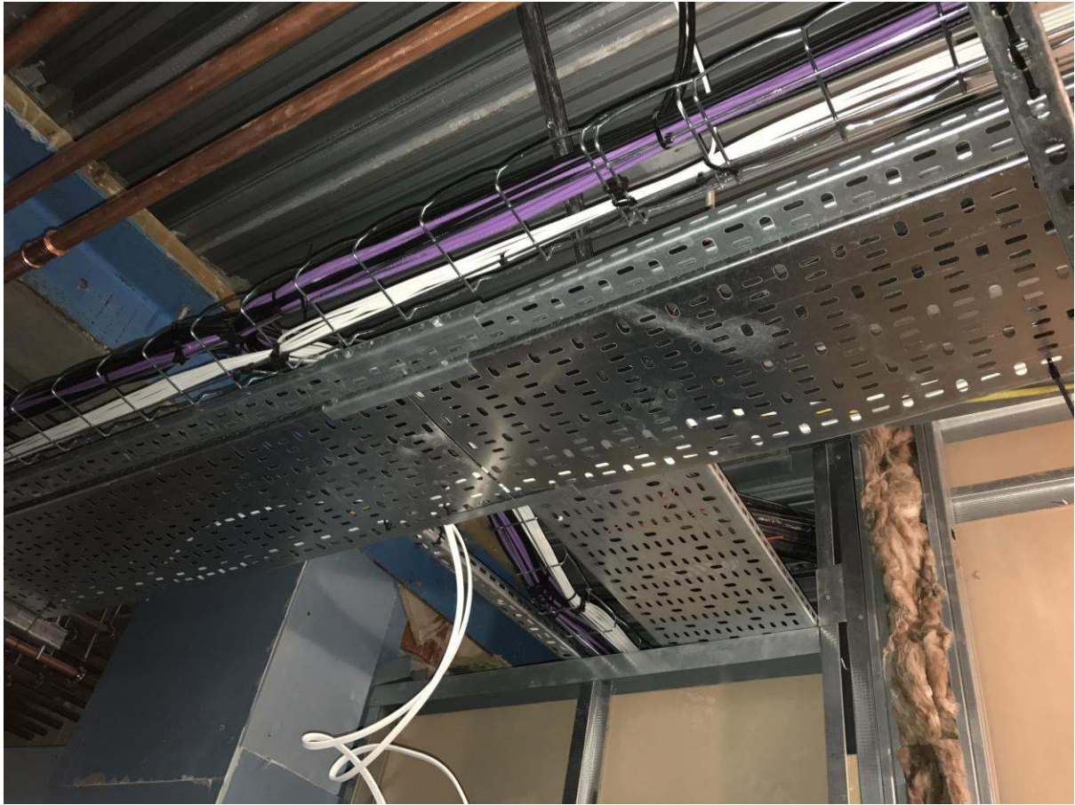
Fifth floor M&E through into stairwell
