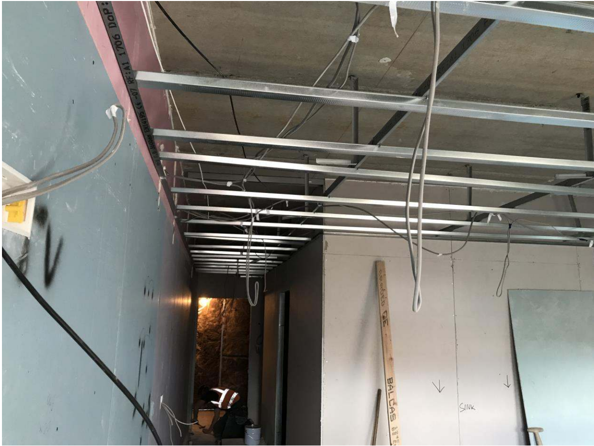
Fourth floor, ready for ventilation ceiling board, plaster
