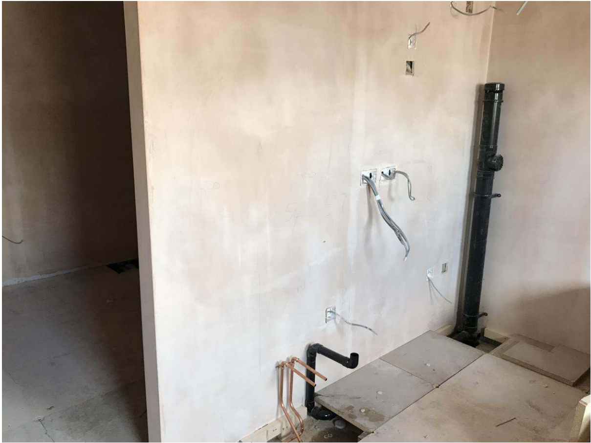
505 fifth floor, fully first fixed and plastered out
