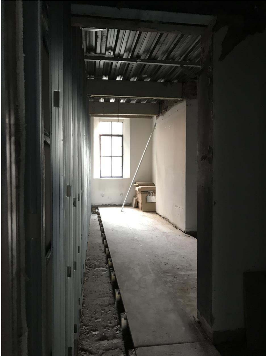
First floor party walls
