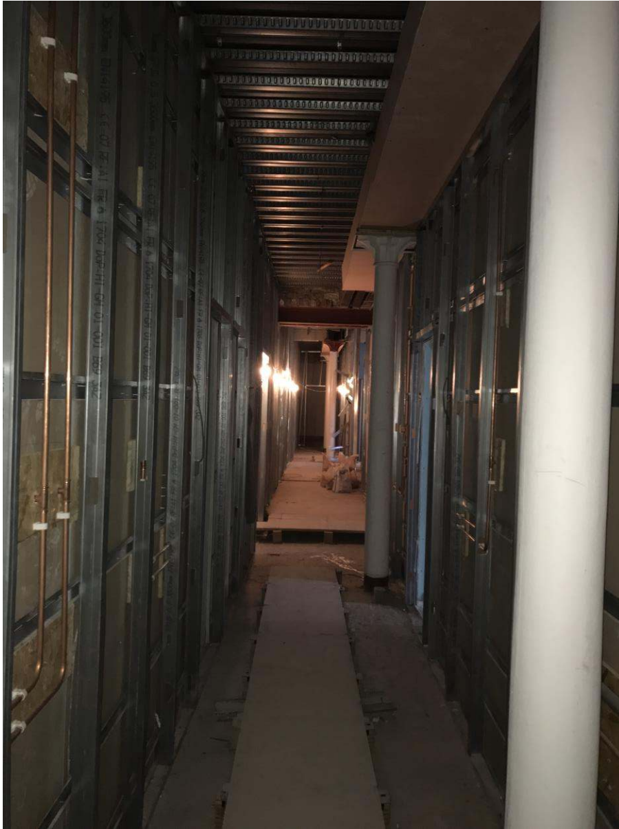
Second floor corridor
