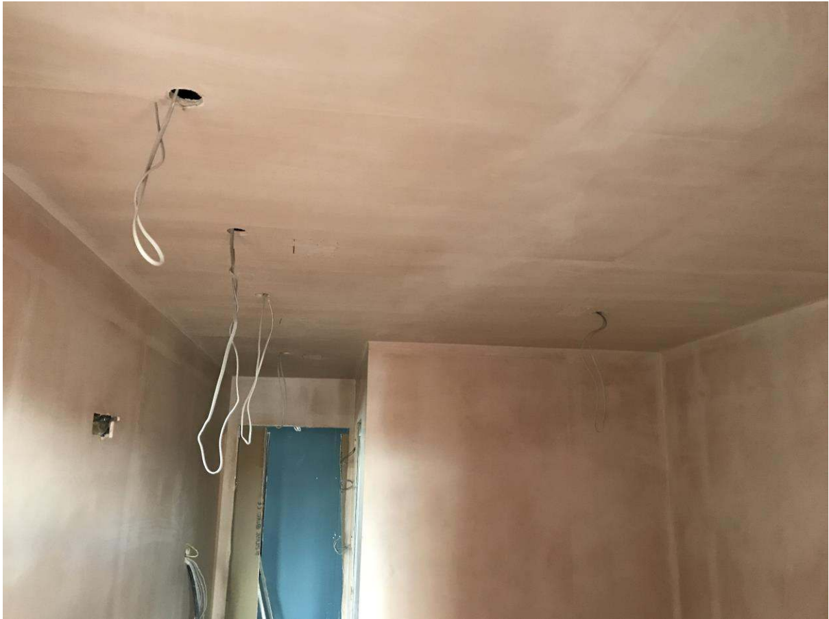
509 fifth floor, living room/hall
