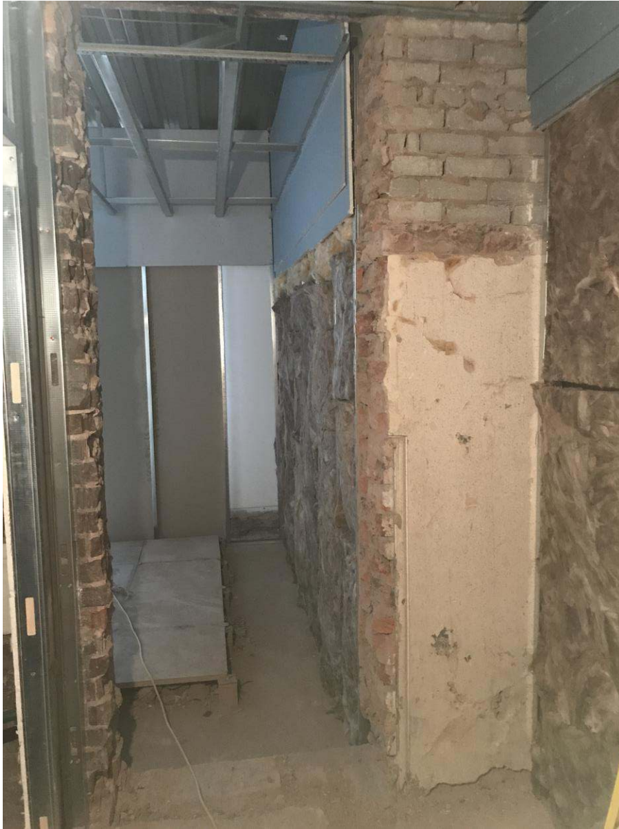
Second floor apartment M&E first fix, party wall insulation
