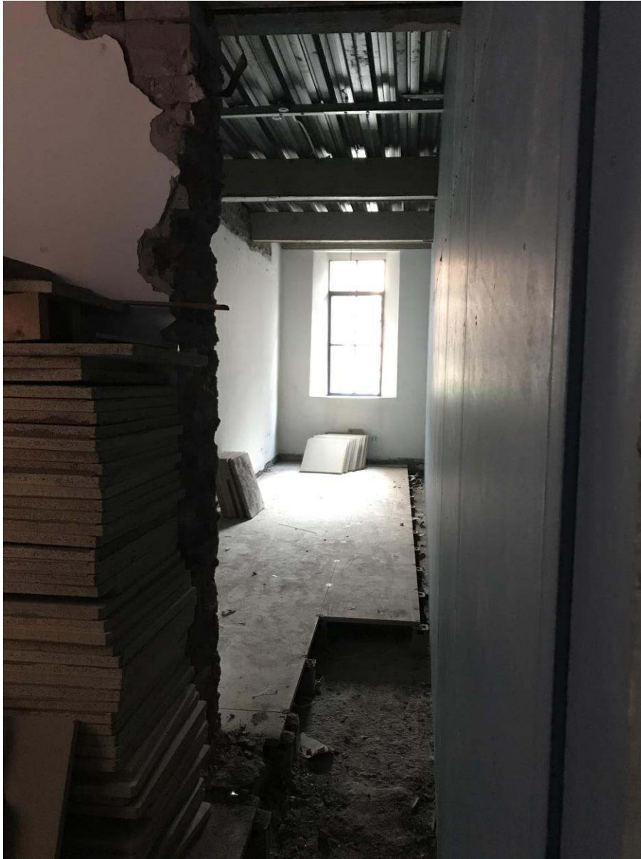
First floor party walls
