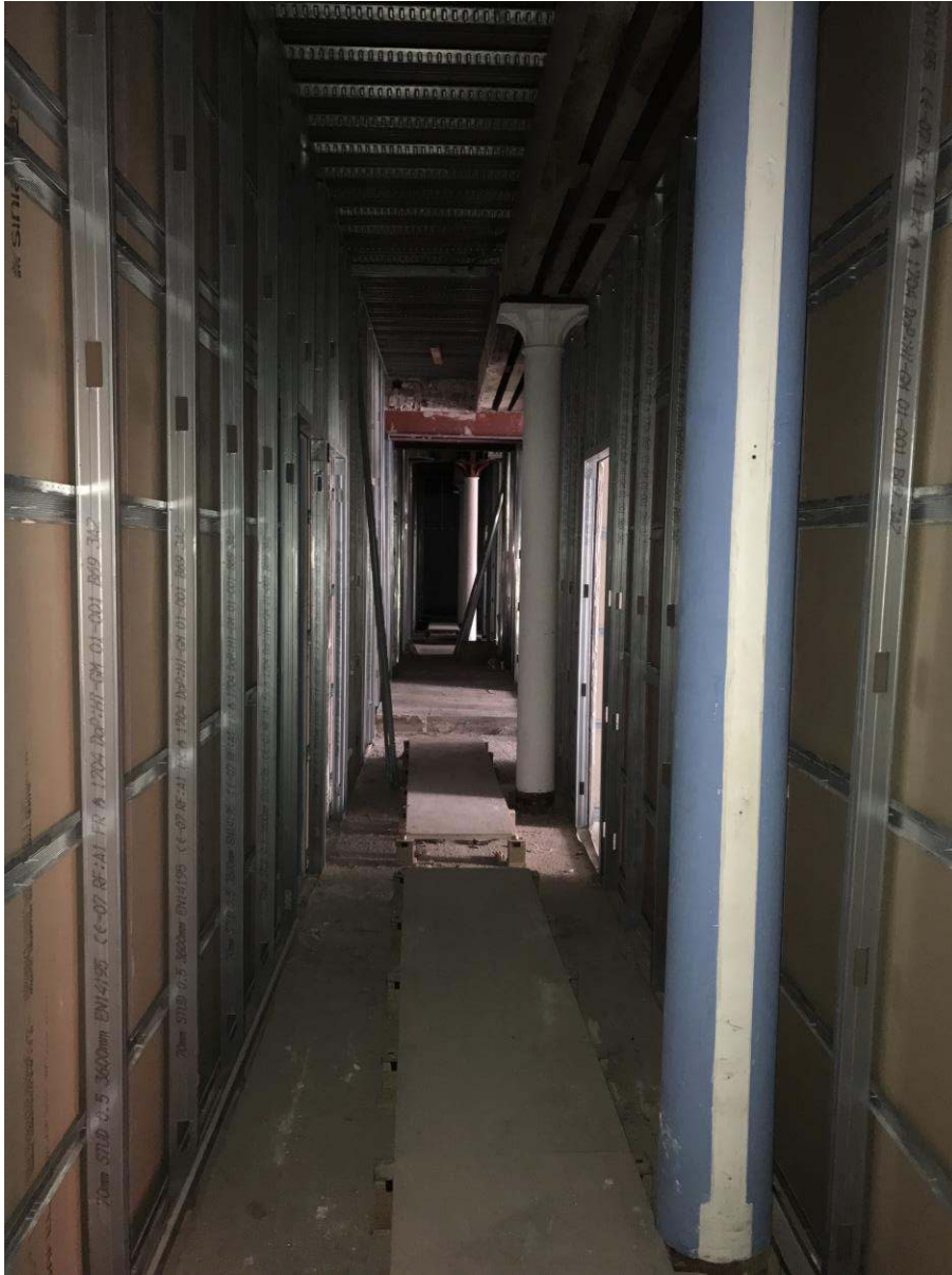
First floor corridor
