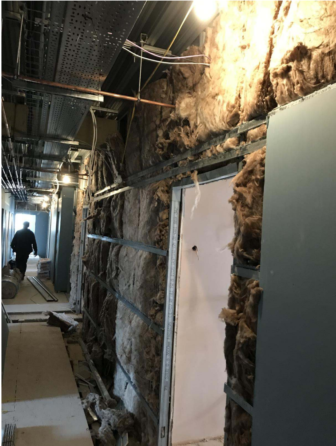
Fifth floor corridor
