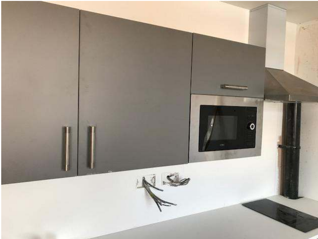
504 fifth floor, setting out kitchen
