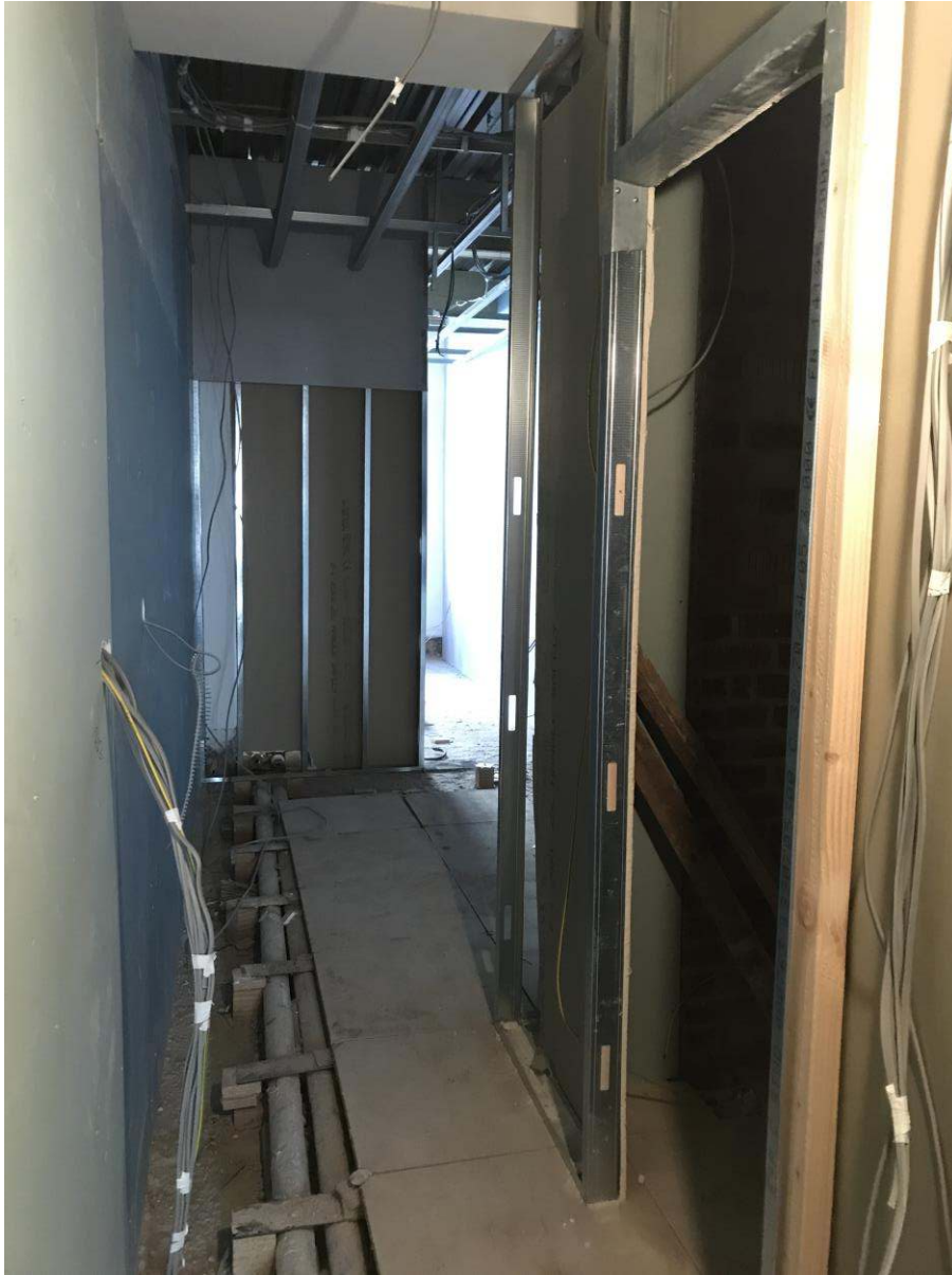
Second floor apartment M&E first fix,
