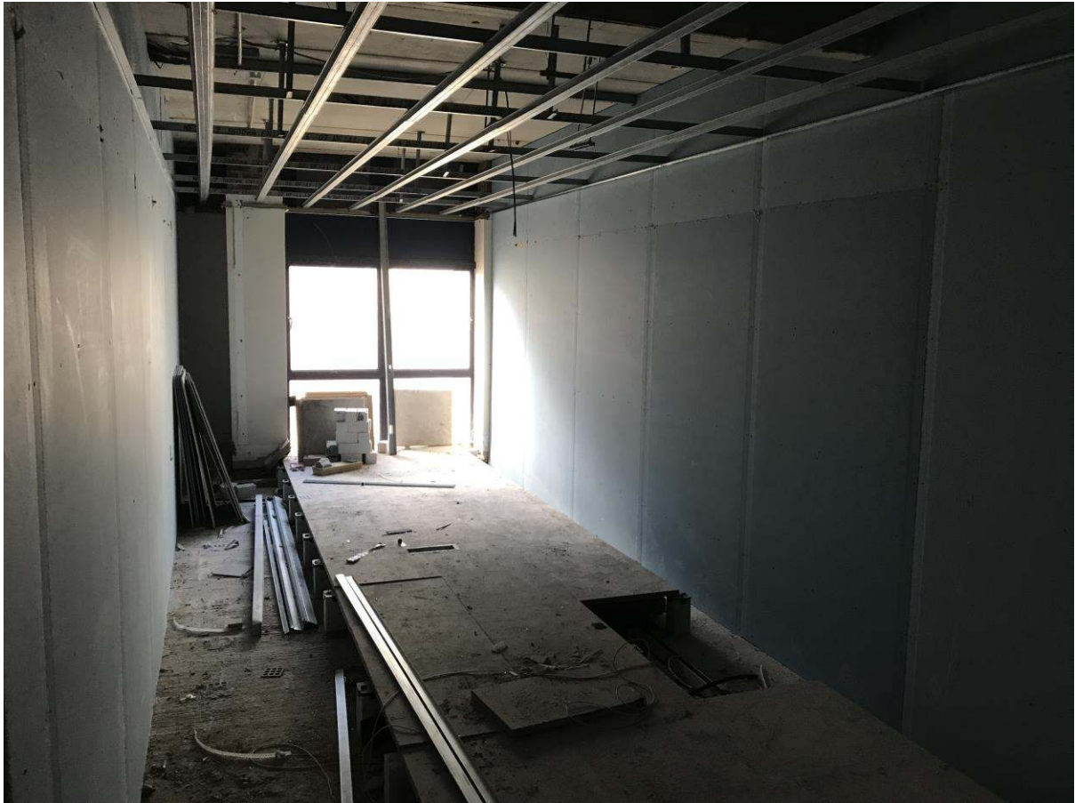
Third floor apartment party walls
