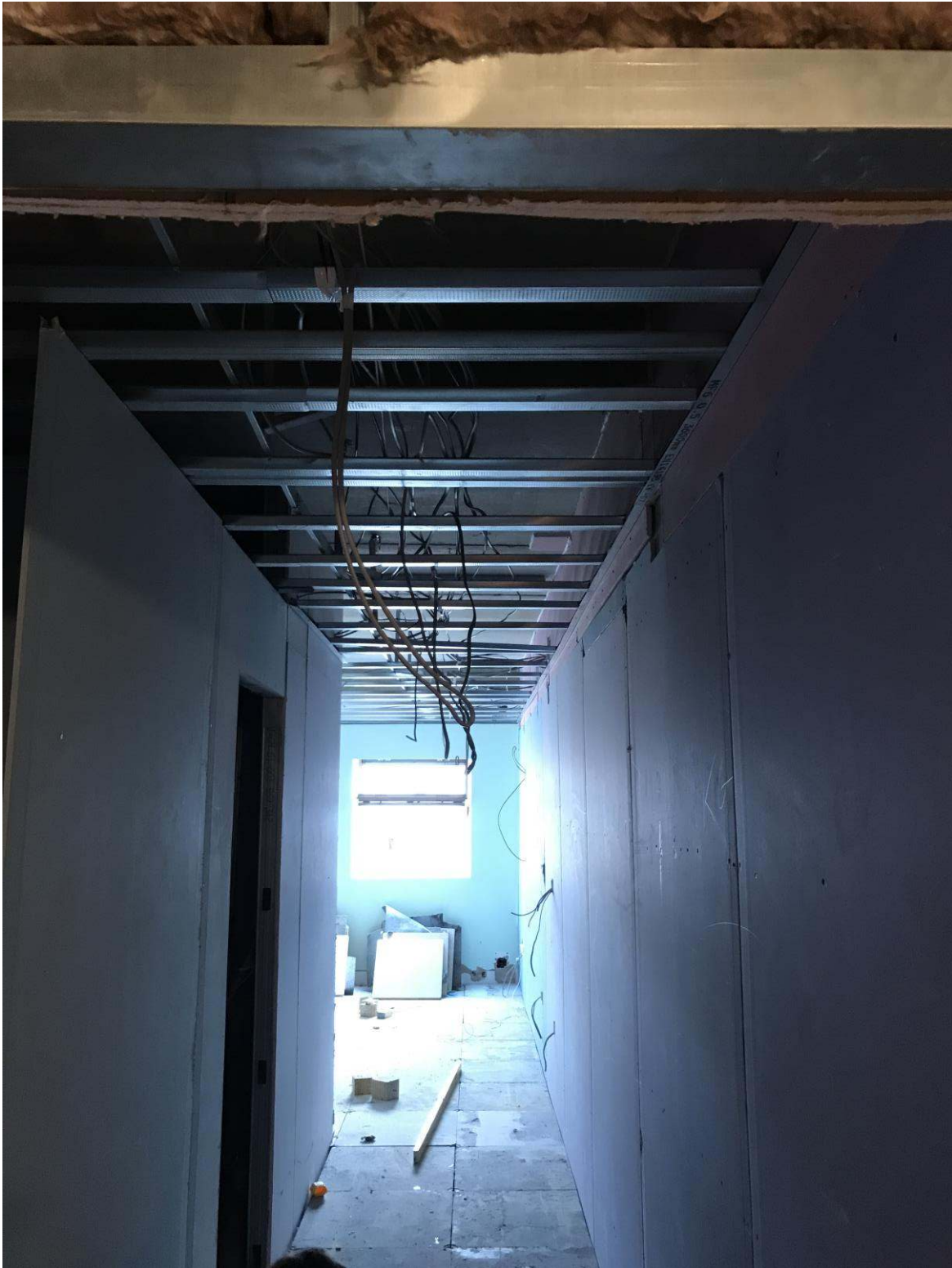
Fourth floor, ready for ventilation ceiling board, plaster
