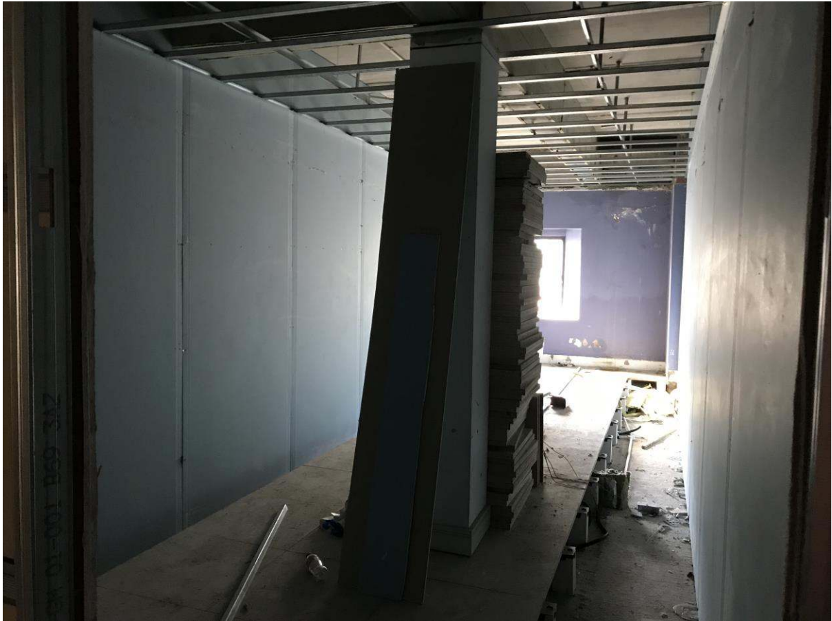
Third floor party walls and ceilings
