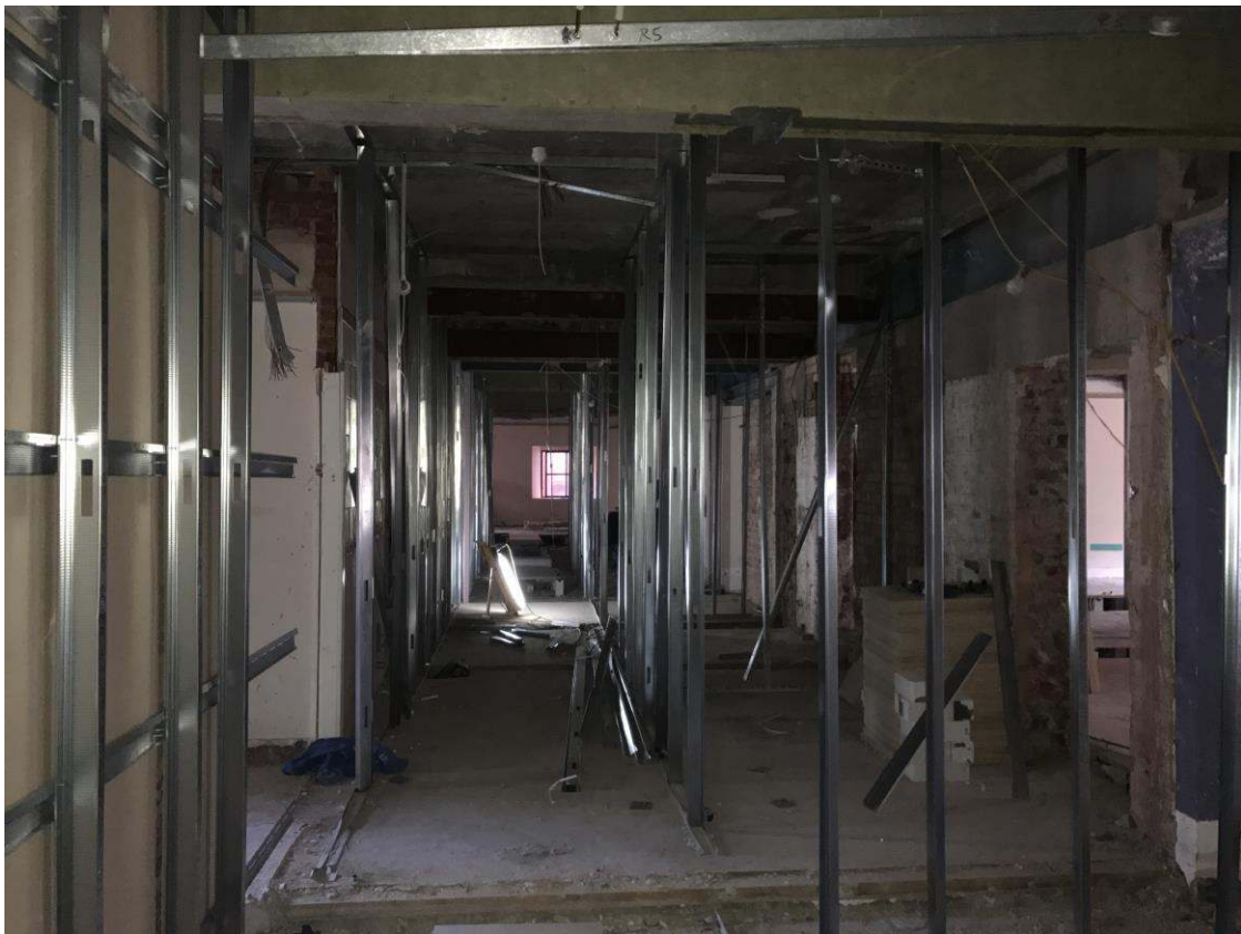
Third floor party walls and corridors
