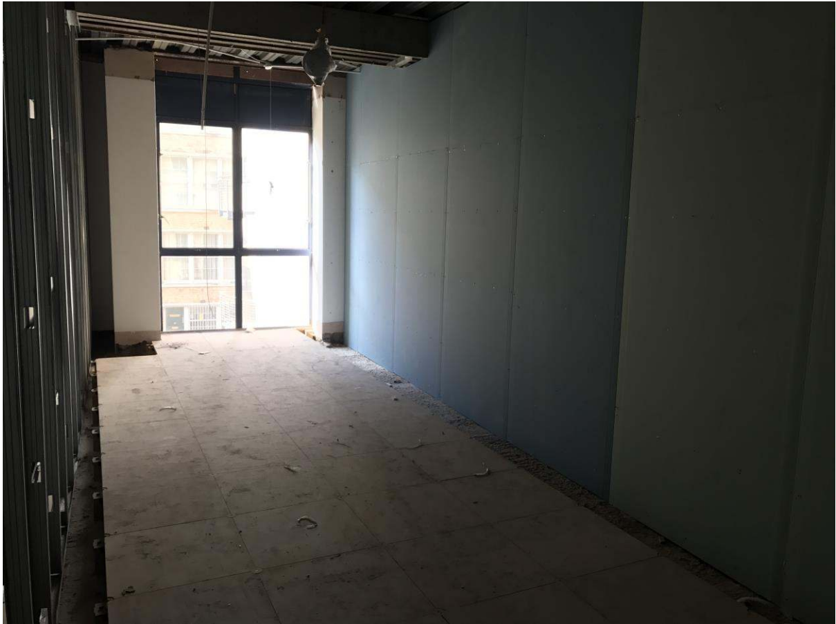
First floor party walls
