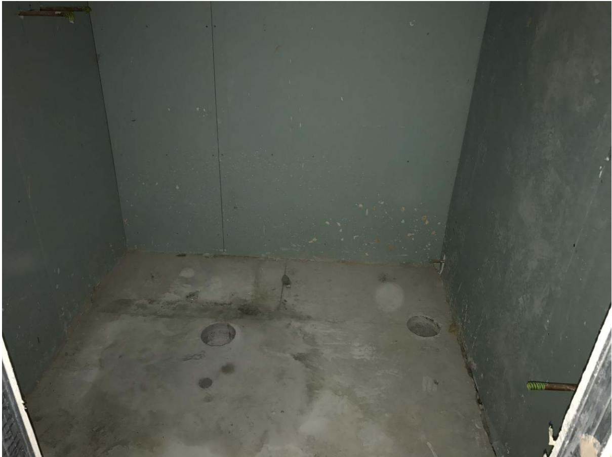
Fifth floor, shower room core holes for drainage
