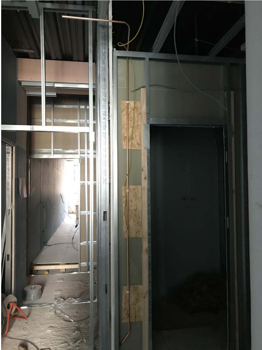
Second floor corridor
