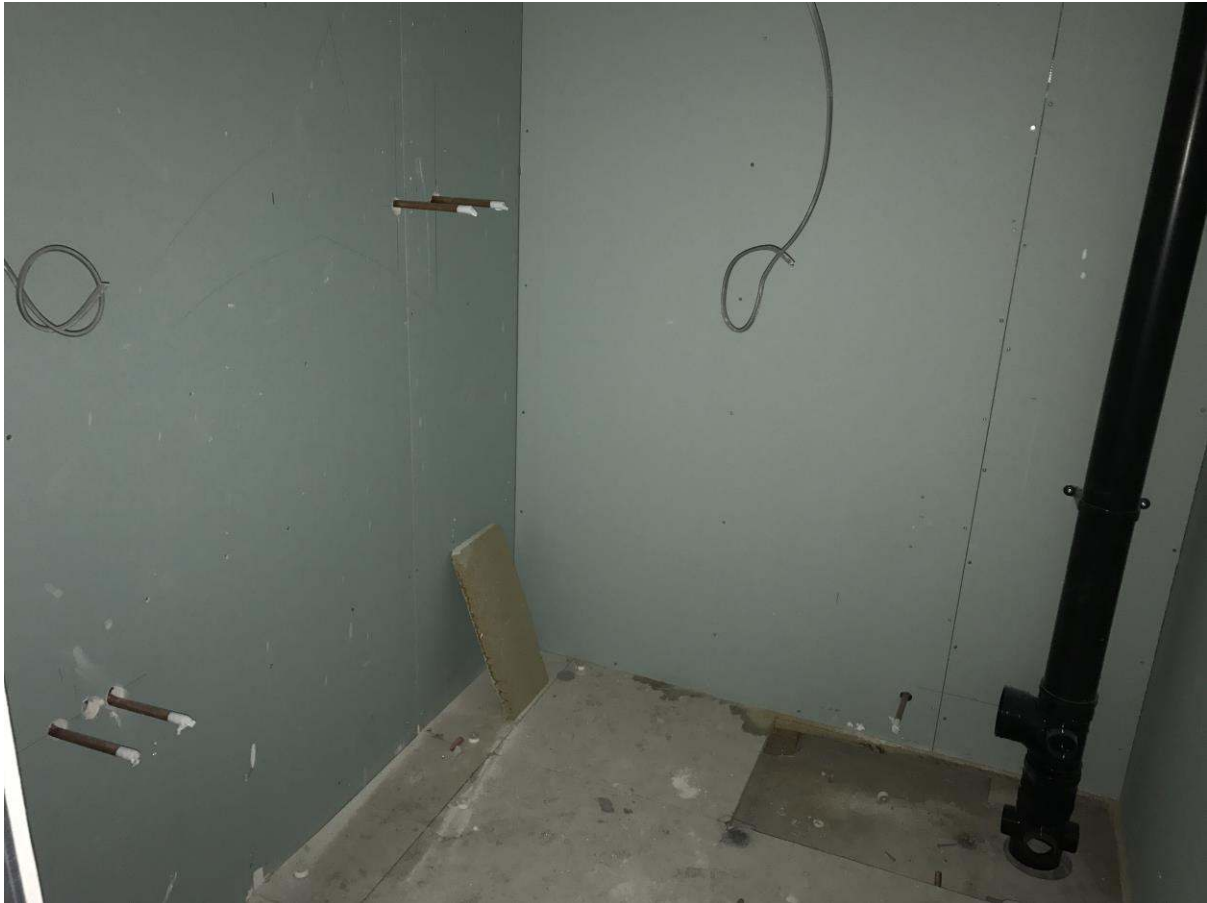
Fourth floor bathrooms fully first fixed, drainage
