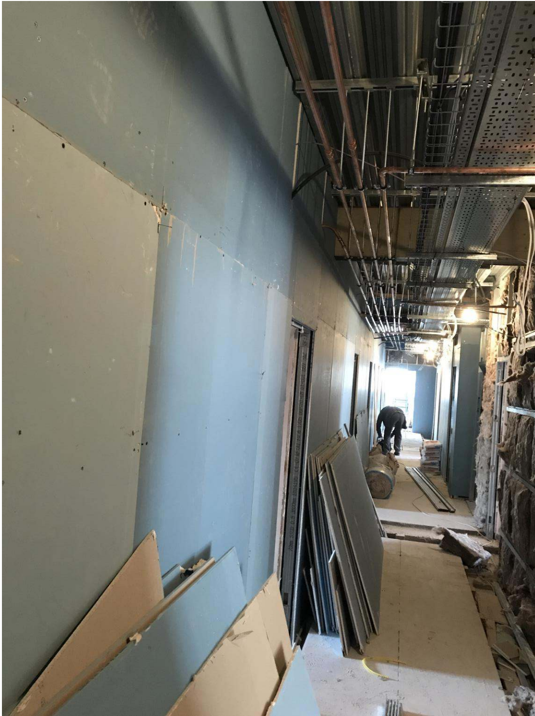
Fifth floor corridor
