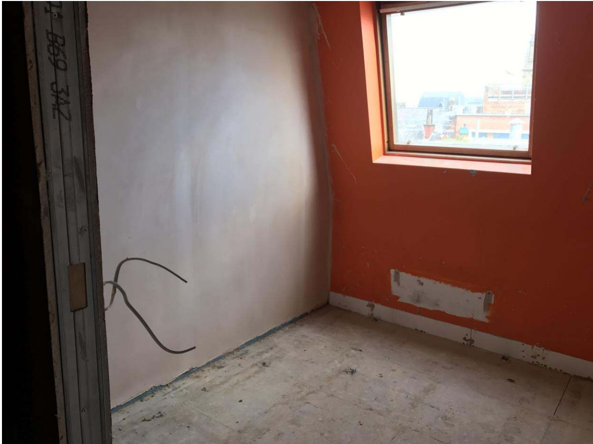
509 fifth floor, bedroom
