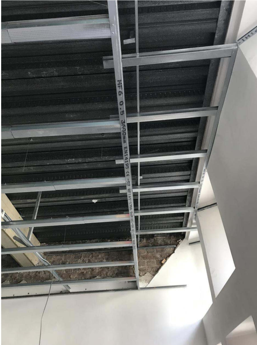
Second floor sample bulk head ceiling on window wall
