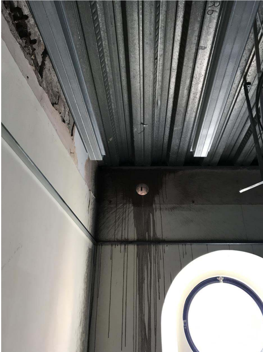
Second floor above ceiling extract vent core holes
