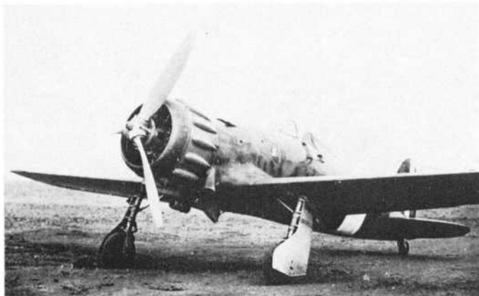
The Macchi MC.200 — also the subject of the cutaway drawing below — was in action early in the North African campaign; its wide undercarriage track, well illustrated in the photograph above, proved valuable during operations from rough airfields in Libya.
