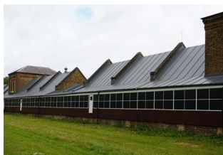
The Royal Gunpowder Mills heritage site had Sika Sarnafil products installed to guarantee a stunning aesthetic and durable roofing solution.
