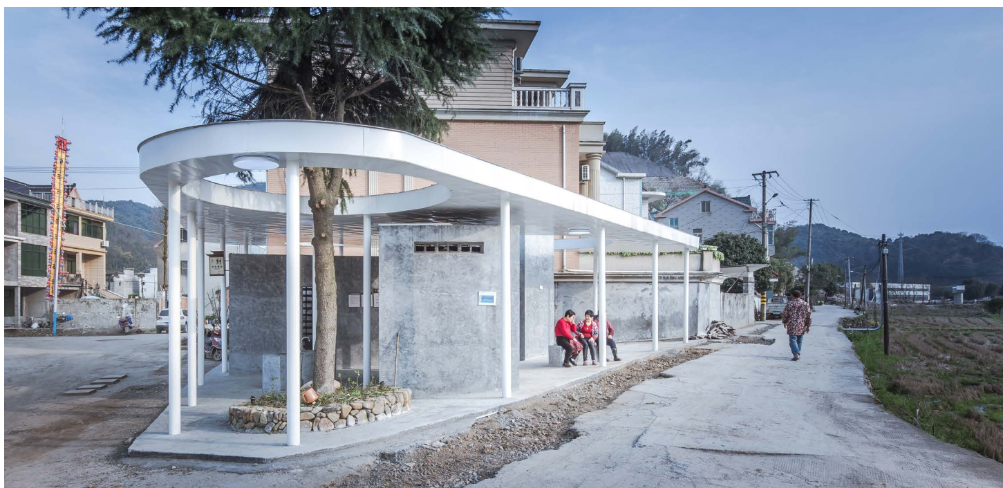
Shulin Architectural Design - Public Toilet at Sanchakou
