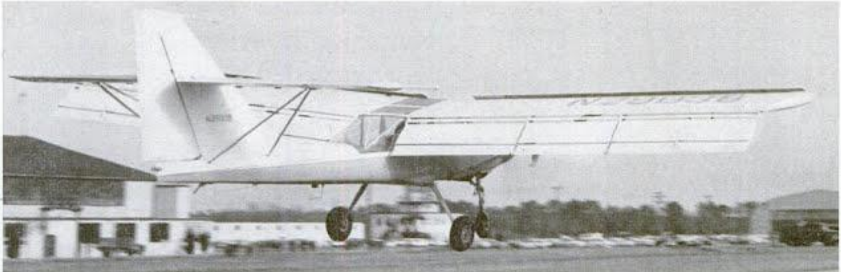
Low-speed flight is achieved by use of slotted leading edge combined with full-span wing flaps in the 4,200-pound gross weight aircraft.
