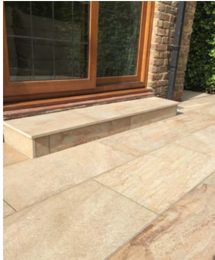
“Fine Porcelain Pointing – Easy with vdw Epoxy Paving Grout”
