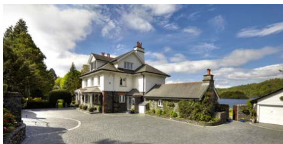
Exposed Burlington Slate Setts Jointed with vdw 850
