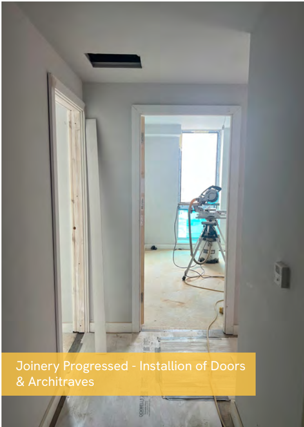
Joinery Progressed - Installation of Doors & Architraves
