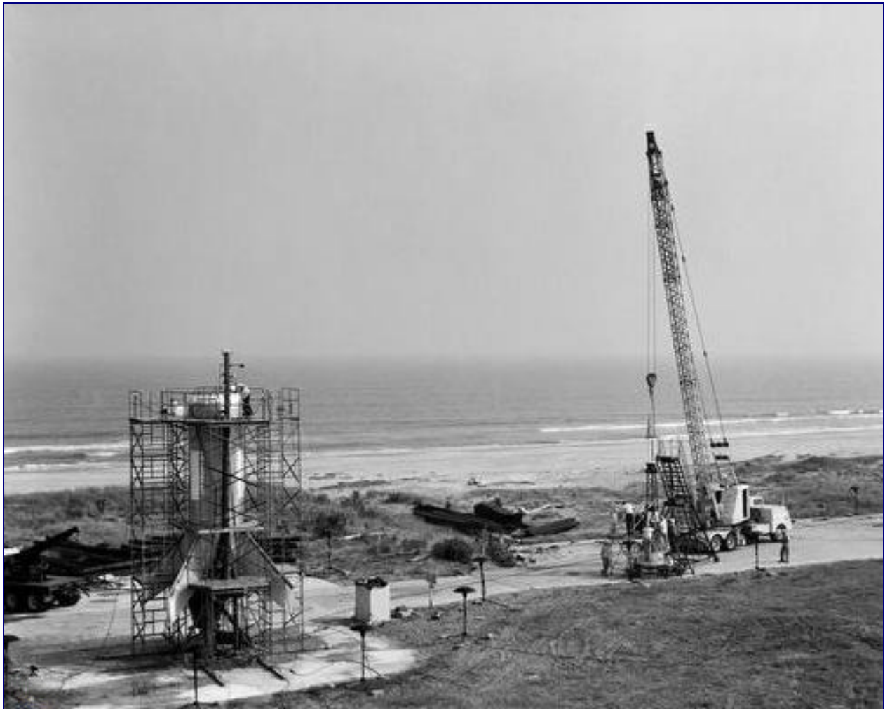
Placing the Little Joe-1 Capsule on its Rocket Booster at Wallops Island, photo courtesy of NASA.
