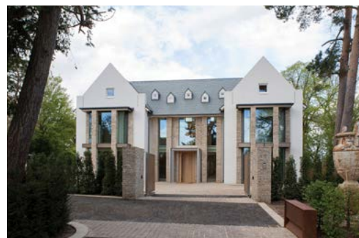
62 Concrete blockwork & Render board materials: Parex Ltd Main Contractor: Optic Realm Ltd, Islington, London Architect: Lees Munday Architects, Gomshall, Guildford, Surrey Rendering Contractor: EnviroREND SE Ltd, Rye, East Sussex
