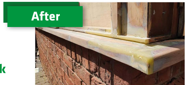
▲ Repair courtesy of DRM Carpentry DRY FLEX® 4 and DRY FLEX® SF used on application
