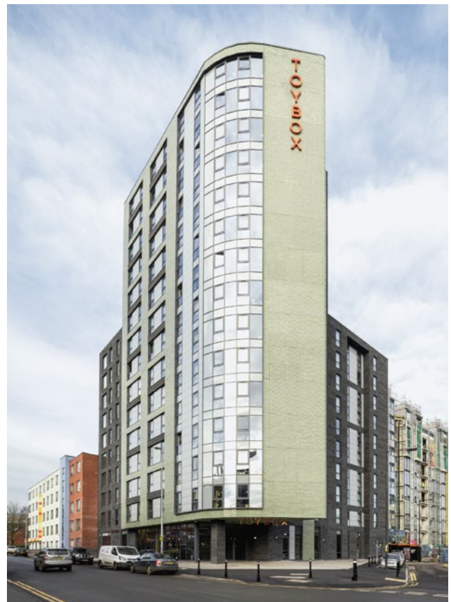
A combination of StoTherm Mineral K external wall insulation system and StoBrick brick slips were specified for the new Toybox student accommodation building in Birmingham.
