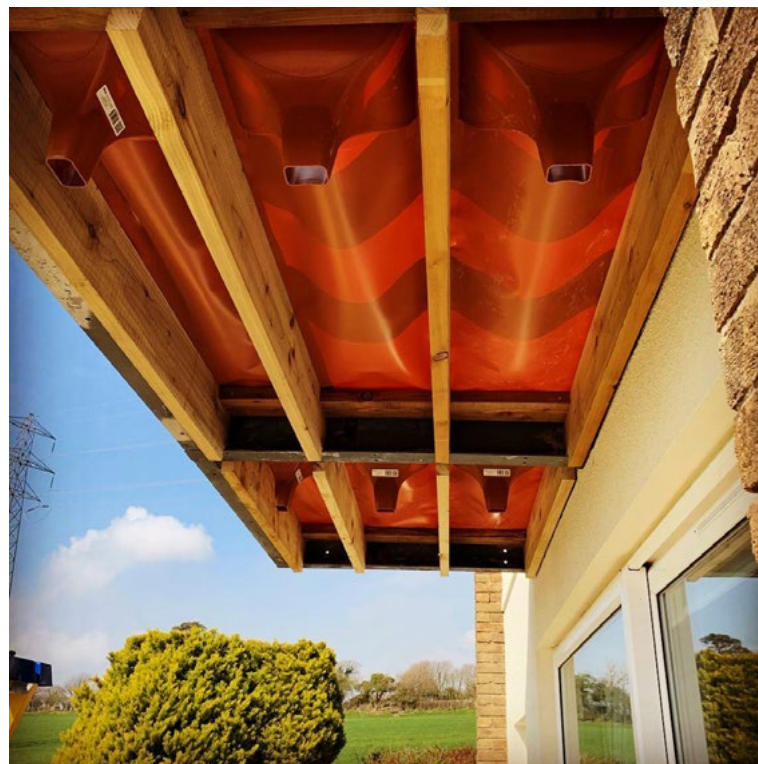
Above, Trex RainEscape installed.
