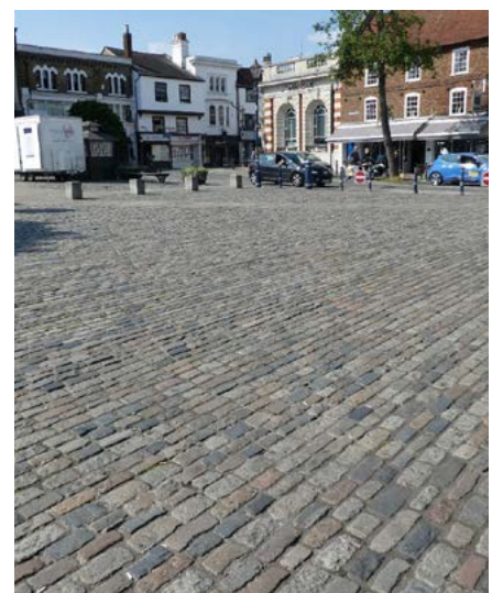
Hitchen Market Square Paving Inspection
