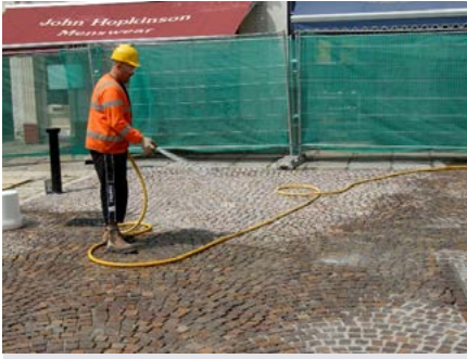
Newark Market Square Installation August 2007: Porphyry setts Thoroughly Prewetted
