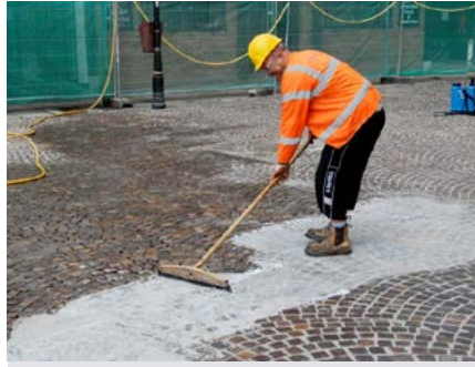
Newark Market Square Installation August 2007: Fast, Ergonomic, Wet Slurry Application
