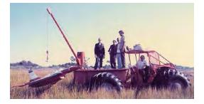
The 0.18-scale drop model being recovered after a successful drop model test at the Plum Tree Island test facility in Virginia. (NASA)
