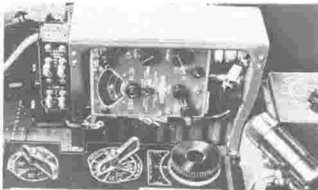
Figure 502 — Radio Compass Remote Control Installed
