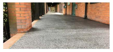
with terrazzo. Different visual effects can be created depending on the size and type of aggregate added at the mixing point to create a bespoke finish.
