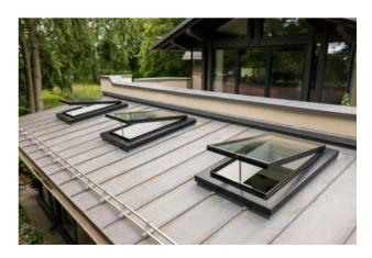
Having whole window U-values of 1.4Wm2K and providing a sleek, frameless finish, the use of a combination of the Conservation Plateau and the neo rooflights from The Rooflight Company were perfect for the job in terms of both aesthetics and thermal performance.
