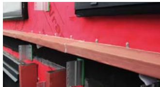
RSM - CAVITY BARRIER FOR RAINSCREEN FACADE SYSTEMS
