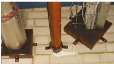
SERVICES THROUGH COLLARS & MULTI PURPOSE BOXES
