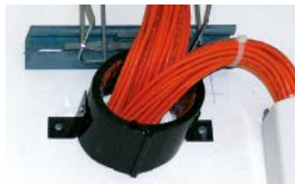
COLLARS CAN BE USED FOR PIPES AND ALSO CABLES
