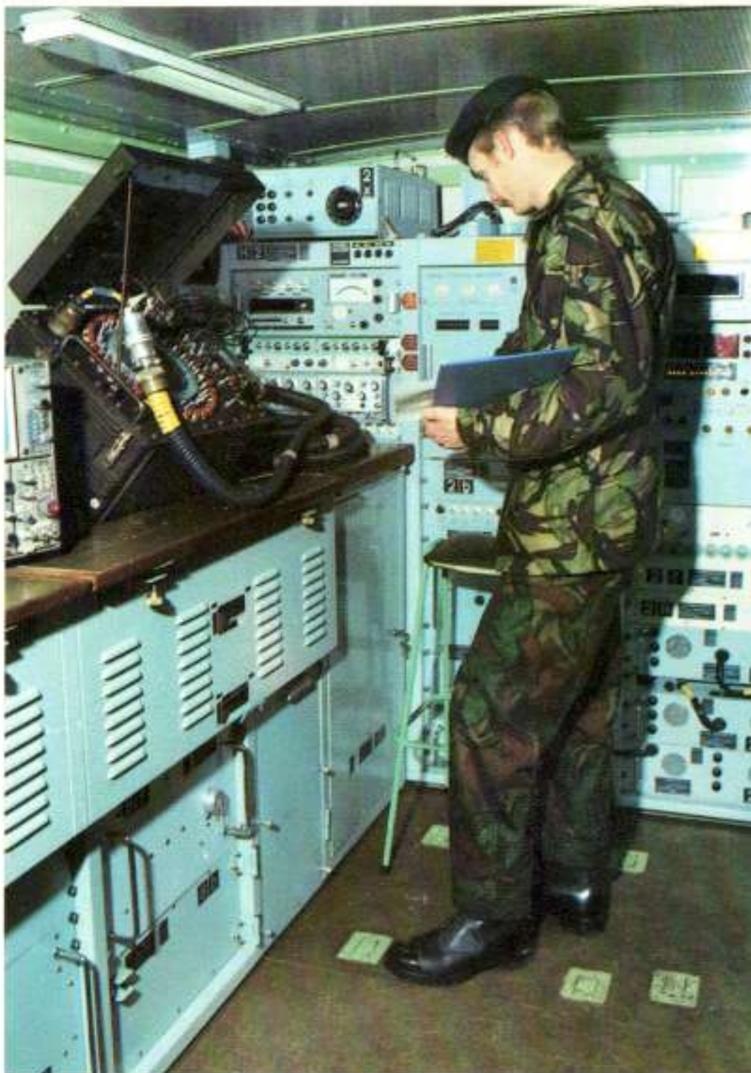
Electronic Repair Vehicle (ERV)
