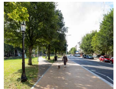
View at VGN showing new path across park, and carriageway reduction to 2 lanes w new footway and mature Elms re-set into extended park lawns © Edward Bishop
