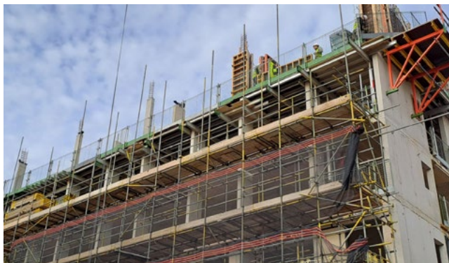
The roof level colonnade beams under construction
