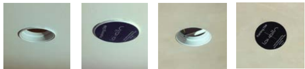
Housing installed Ready for plastering After plastering Ready for painting
