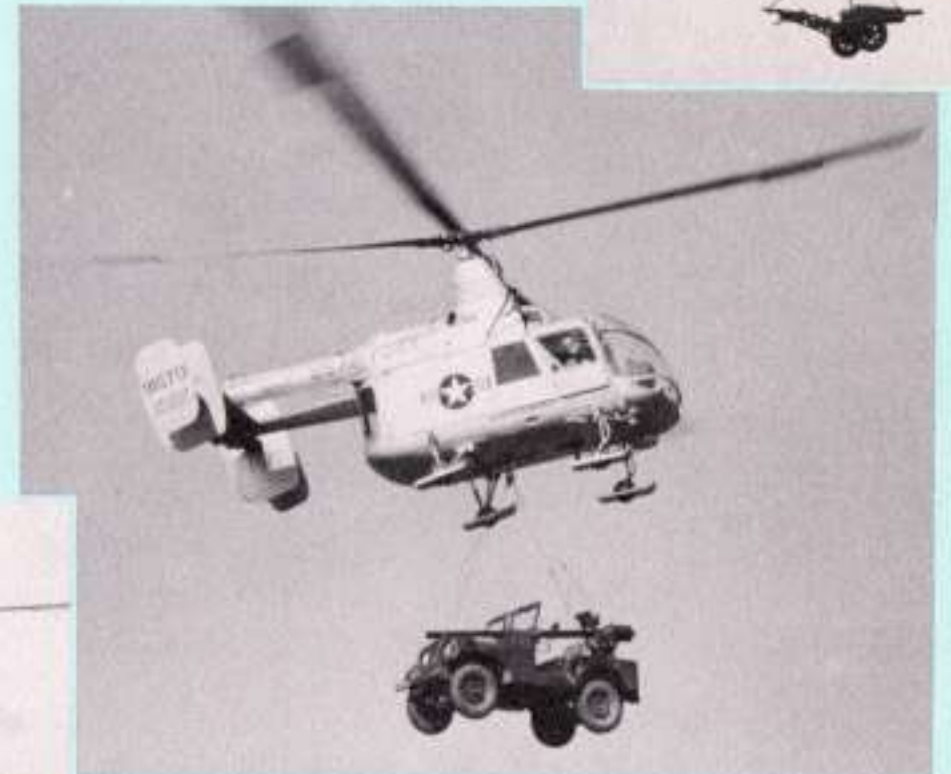
transporting 3400 lb. jeep-mounted 105mm recoilless rifle . . .
