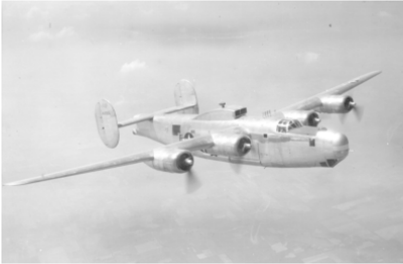
The B-24 Flying Laboratory, shown in flight in July 1946, specialized in aircraft icing phenomena. Operating from its home base at the NACA's Cleveland facility, the military aircraft tested the cold weather endurance of jet engines subjected to freezing flight conditions. The scoop atop the fuselage sent combustion air (moistened by water nozzles) to a turbine engine mounted in the B-24's bomb bay. (NASA Photo Number C-15318.)
